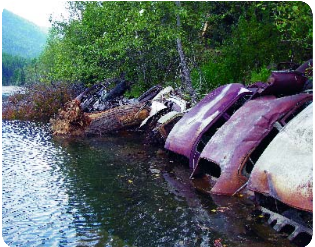
Car bodies, from the 1940s and 1950s, were used to protect the river bank. The work this summer included adding a large tree trunk and root wad.
